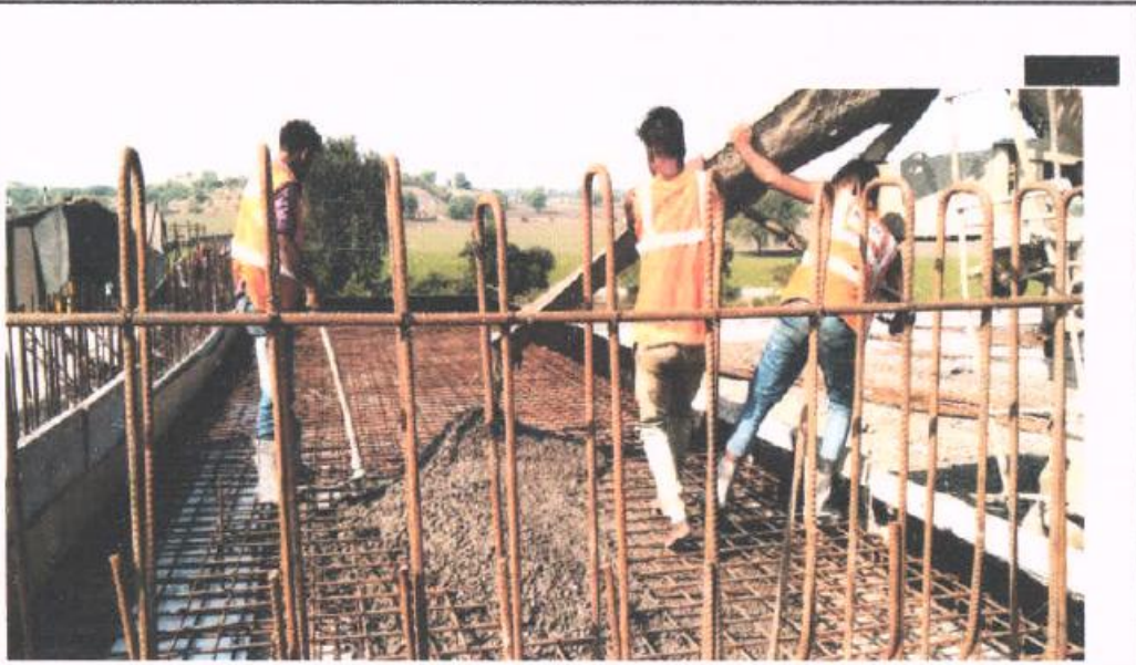
VUP at Km. 12+125 Concrete pouring work for Terminal slab A1 side LHS
