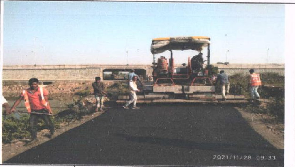
Km. 37+053 (Junction) Laying of Bitumen Concrete 1 st layer in progress RHS
