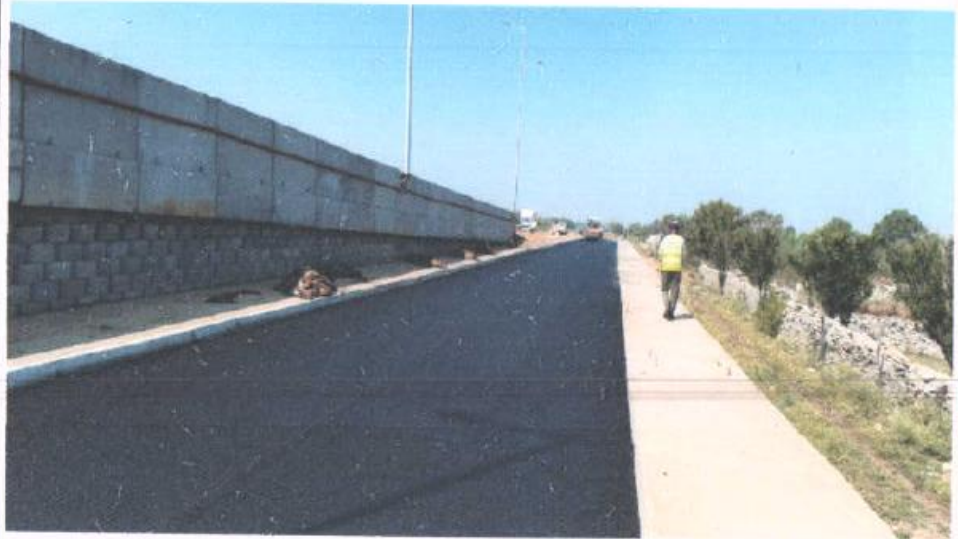
Km. 17+000 Laying of Bituminous concrete (BC) LHS
