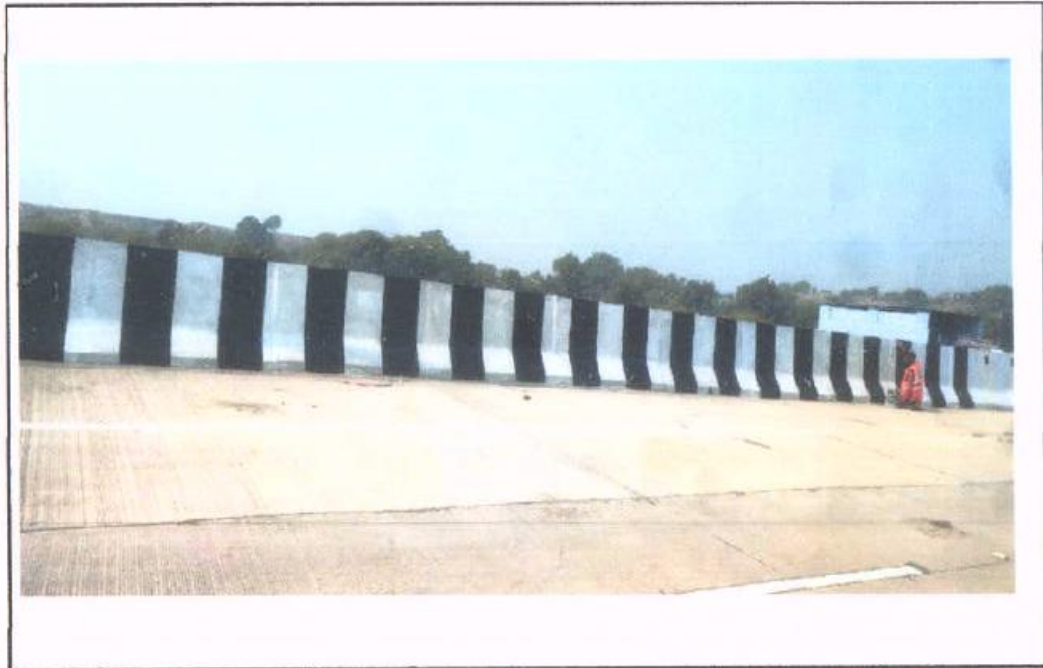
Km. 21+183 Painting work of crash barrier RHS
