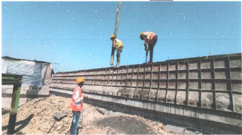
VUP at Km. 12+125 Concrete pouring work for Terminal slab A1 side LHS
