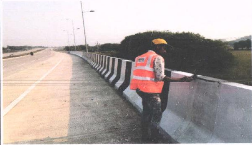
Km. 21+183 Painting work of crash barrier RHS
