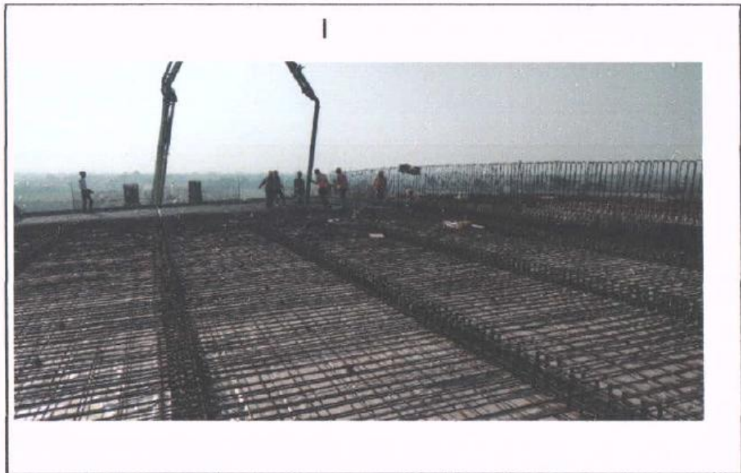
ROB At Km. 44+158 Concrete pouring work of slab P1-P2 BHS
